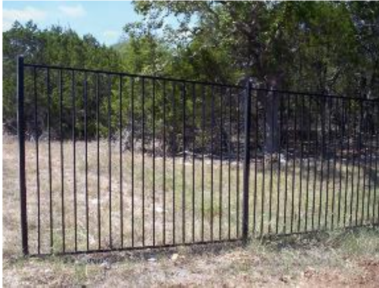
Figure 10. Wrought Iron Fencing
