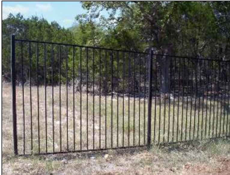
Figure 10. Wrought Iron Fencing
