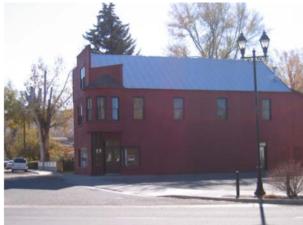
Figure 2 Brick Store (former IOOF Hall)
