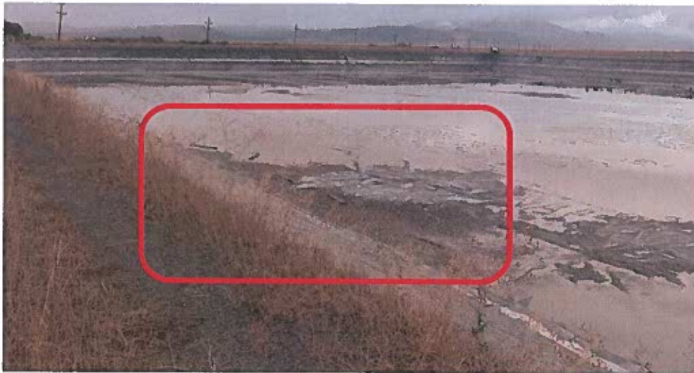
Figure 3: Ballasts lying along the edge of the south pond perimeter on October 4, 2018.
