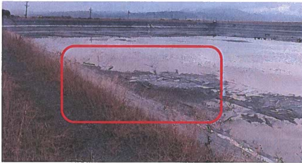
Figure 3: Ballasts lying along the edge of the south pond perimeter on October 4, 2018.
