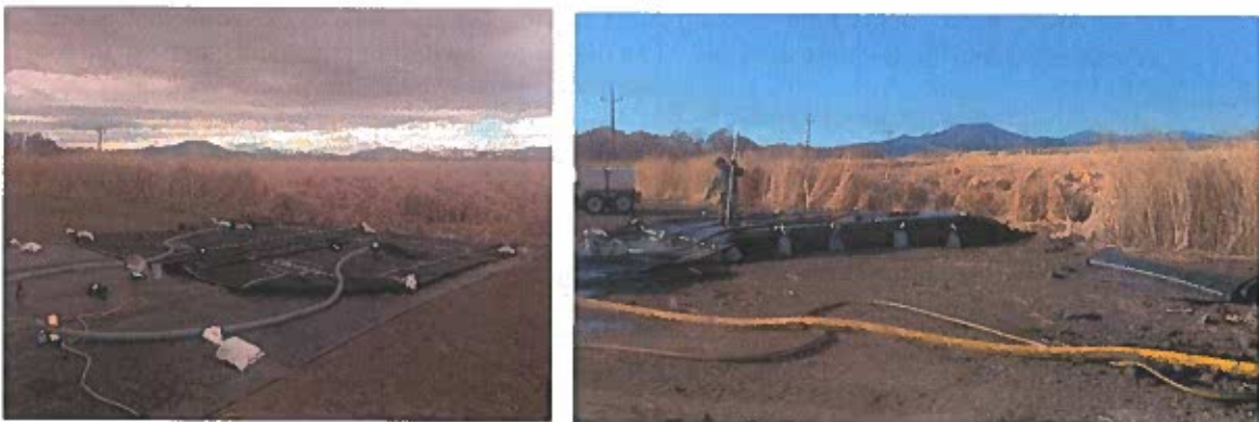
Figure 1: Geotubes currently present at the WWTP. Left shows the empty geotubes before the desludging activities took place on the south pond in November 2019, right shows the geotubes filled with sludge and seeping water during the desludging of the south pond. These geotubes will be utilized to desludge the north pond in September 2020, if needed.
